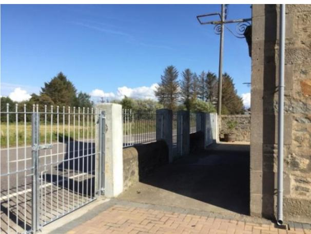
The refurbishment of Boharm Hall has continued with replacement of the railings and gates and re-pointing of some of the walls around the car park.
