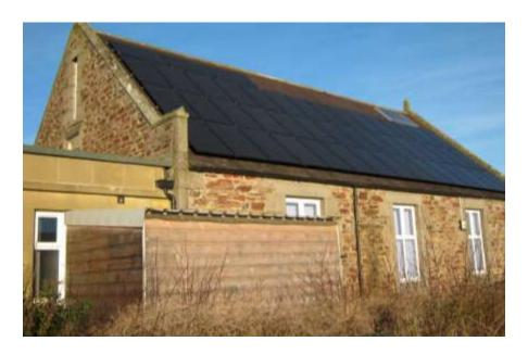
"The grant contributed to a solar panel array at the Newmill Hall. This complements our biomass boiler as some of the electricity is used to power the electric pumps which the boiler requires.
