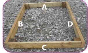
5. Start about 5mm lower on the board that will form the corner with this board, so the screws don't meet each other in the corner post.
