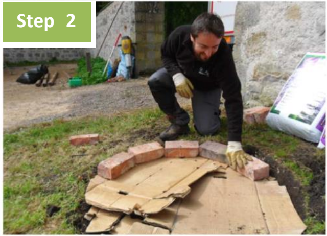
Lay cardboard down and place bricks on top.
