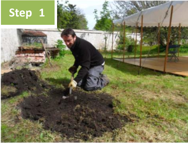
Level the ground.
